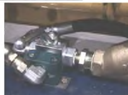
Remove the hose connection and drain the oil from here for 30 minutes
